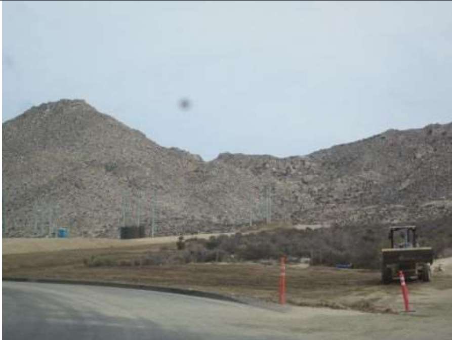
Photo 5: Topsoil was observed being distributed where temporary trailers were staged at the ECO substation in accordance with MM-BIO-1d.
