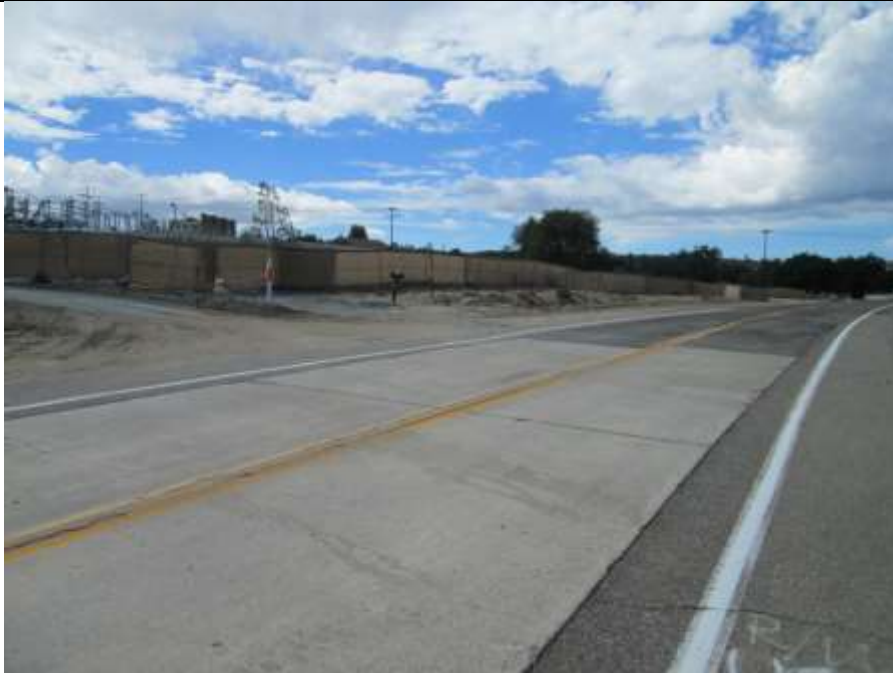
Photo 6: At the Boulevard Substation rebuild site, the point of ingress and egress connecting to Old Highway was observed free of sediment track-out in accordance with the SWPPP and MM-HYD-1. Additionally, in accordance with MM-VIS-3a, the perimeter security fence's screening material was observed intact upon repair.
